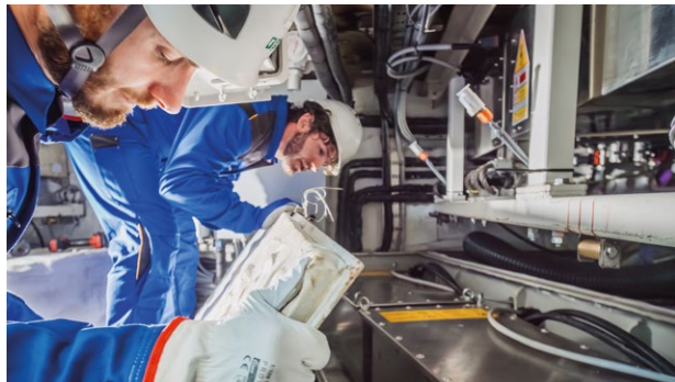
The Hybrid Architect Team during the installation of the salt batteries
