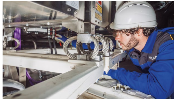
Wire rope mounts are installed to preserve electronic components on board.
